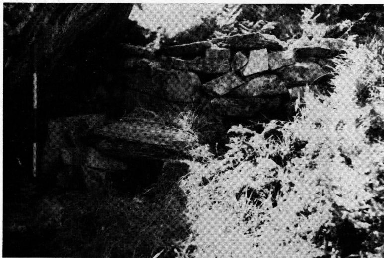
(2) From outside, showing the flue end.
