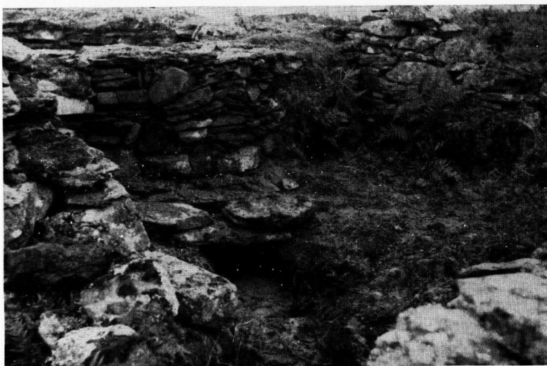
(3) From the N.E. entrance, after reconstruction of the outer side of the bowl arc and the outer end of the flue. The stepped flue base is as excavated.
